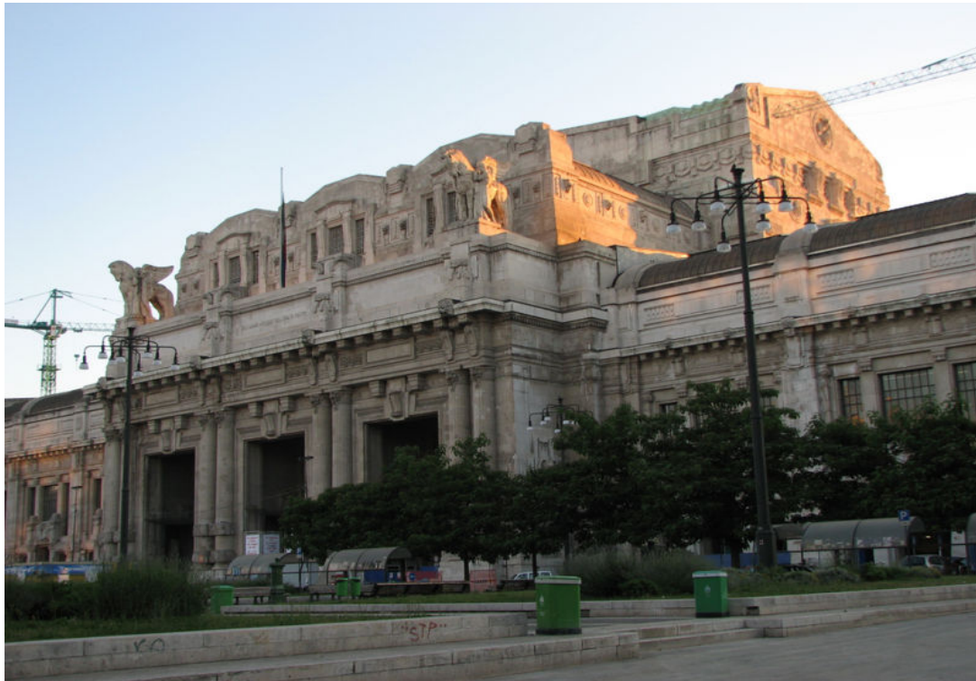
Milan Central station
