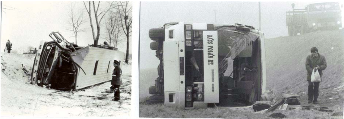
Fig.5. Strong superstructure assures the survival space
