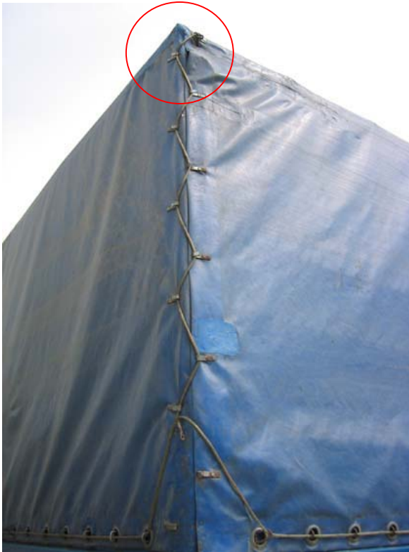
A: No thong - only elastic rope and hooks. Note that the rope does not even match in length. (Rear view of the truck).
