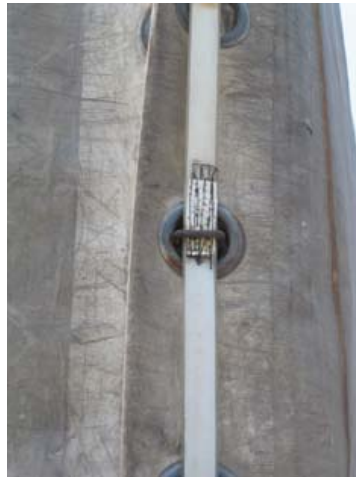
B: Thong repaired or joined with an extra layer of textile and sewing.
