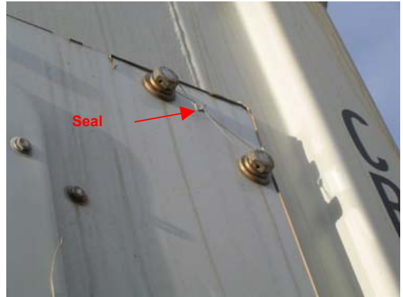
B: Upper part of the frame, bolts and seal for the refrigerator unit.
