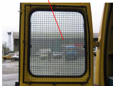
F: Rear door - window secured by metal gauze.
