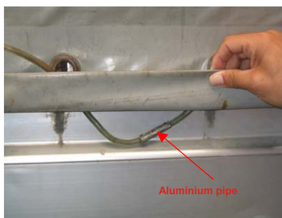
D: TIR-wire jointed - a piece of aluminium pipe being used.
