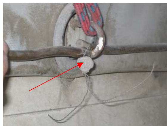
D: Rather unusual joining of a broken or cut wire. Jointed behind the cabin with a CUSTOMS SEAL.
