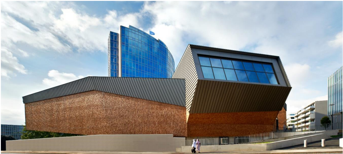
Fig. 5 and Cover image This sculptural timber building contrasts strongly with the glass and steel of the surrounding buildings. By choosing the sustainable renewable resource wood as the main construction material, the client highlighted its commitment to sustainability.
