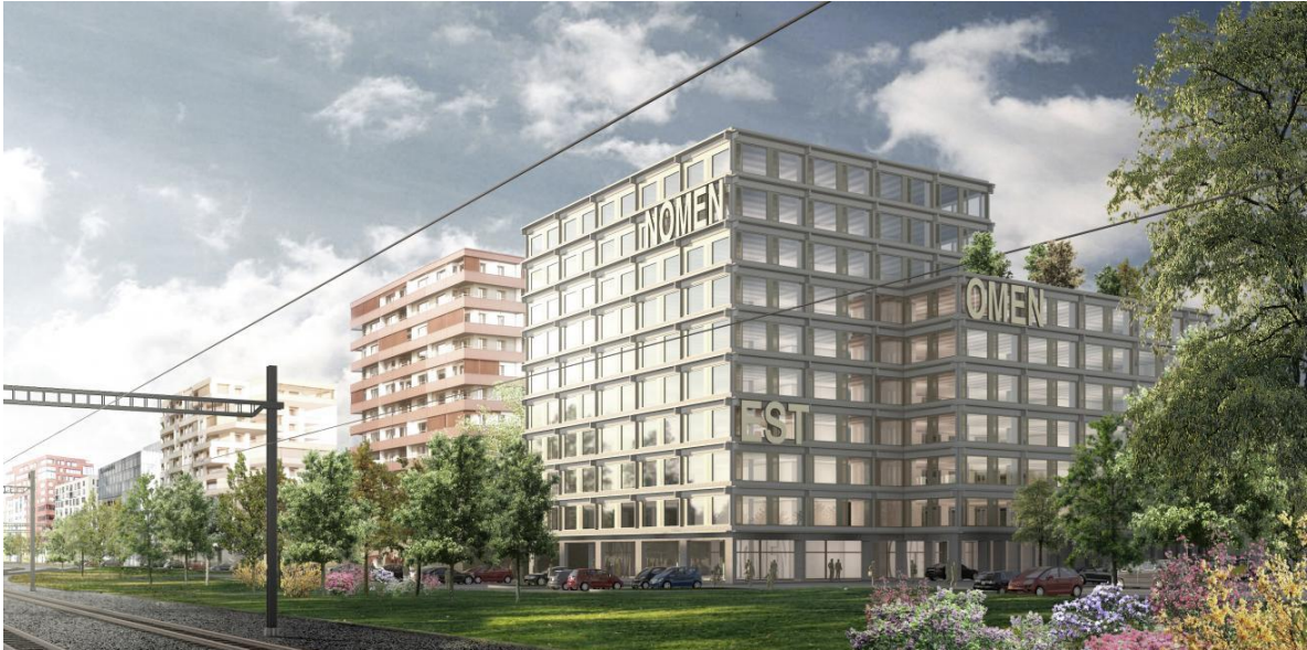
Fig. 1 Right, Switzerland's first ten-storey wood-concrete composite high-rise
