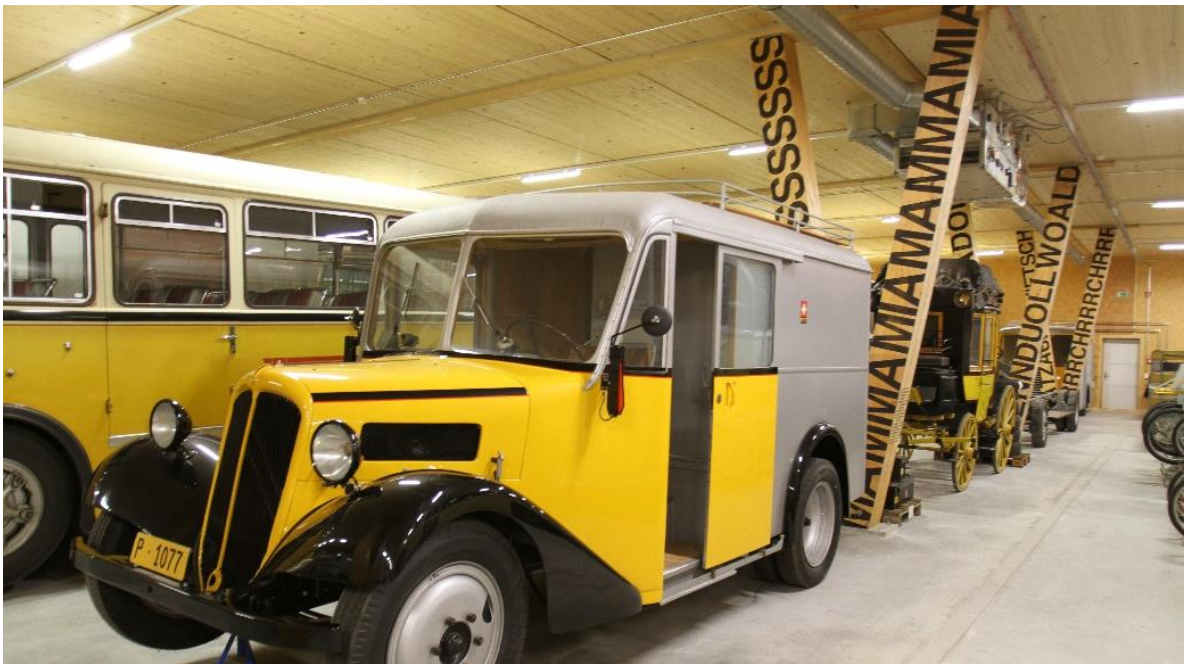
Fig. 9 The appearance of the interior halls is characterised by the V-shaped supports and ceilings constructed from stacked timber elements.
