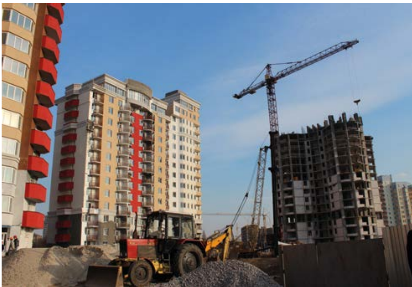
Picture 9. A social housing under construction
