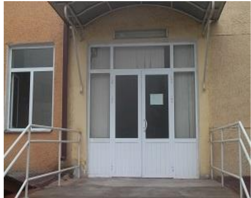
Entrance to polyclinic for which thermographing was carried out
