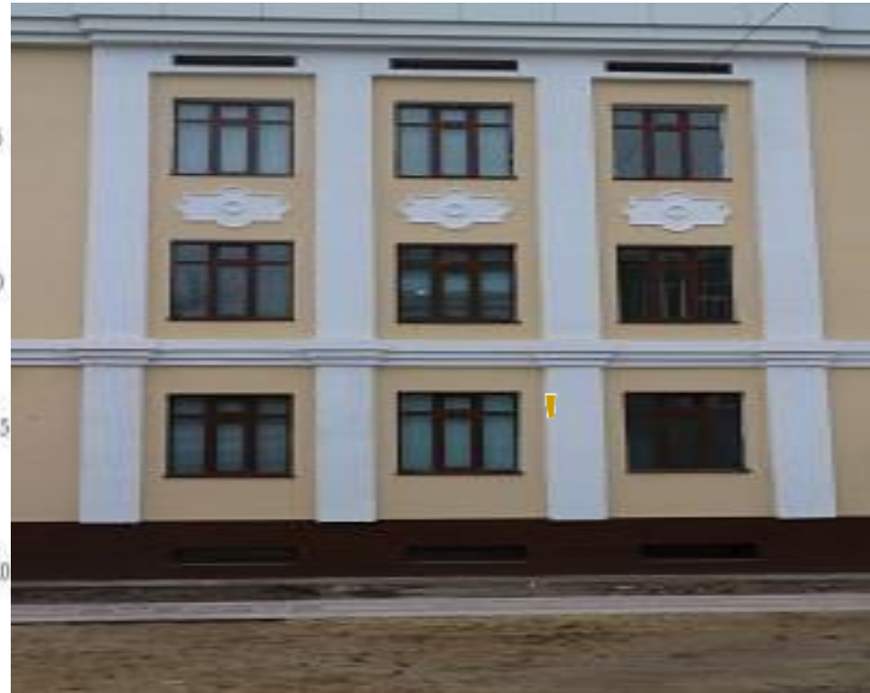
Fragment of the facade for which thermographing was carried out
