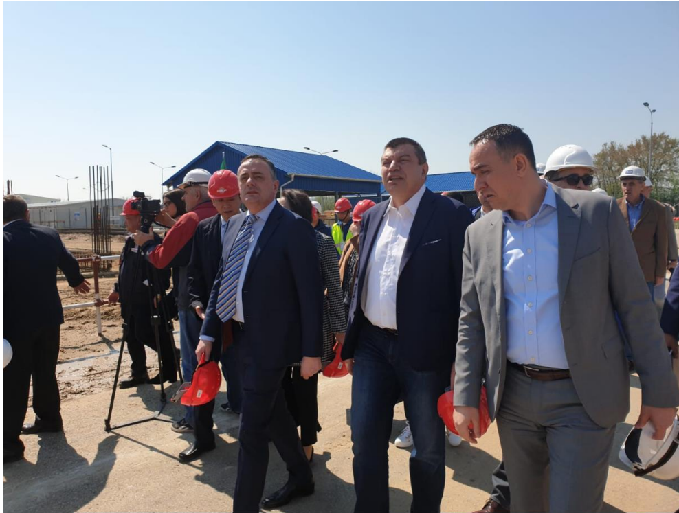
The above pictures shows the Minister walking over the Kostolac B3 site, construction works clearly visible on the left side of the picture.
