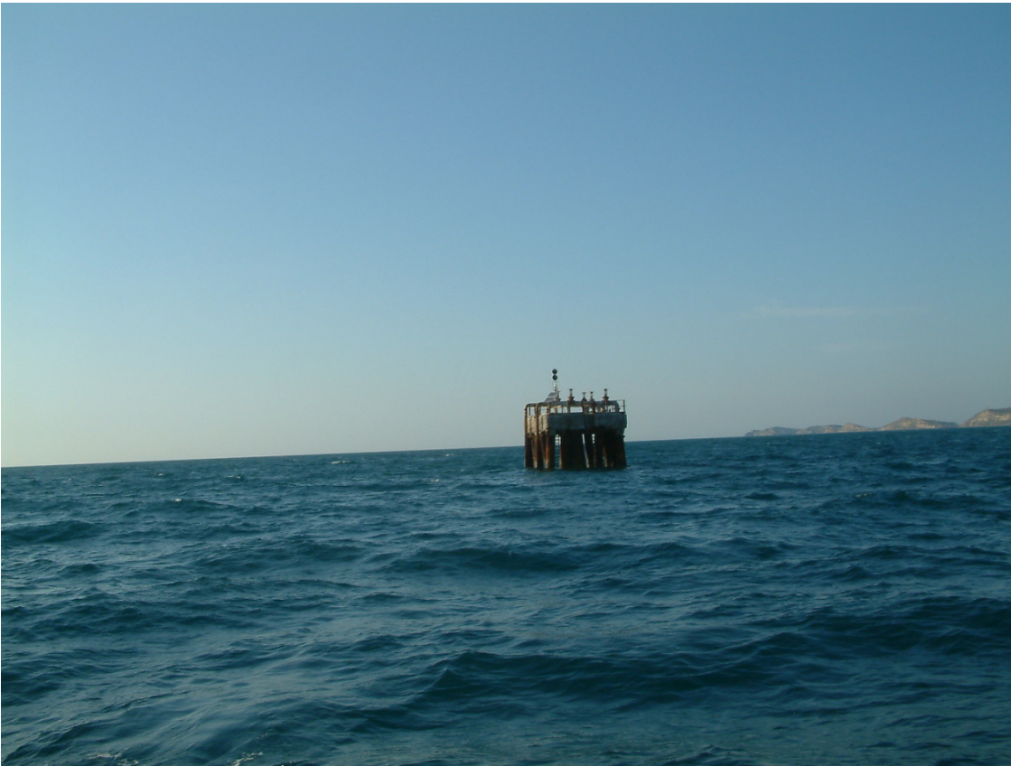
The single mooring point in the on-shore area.
