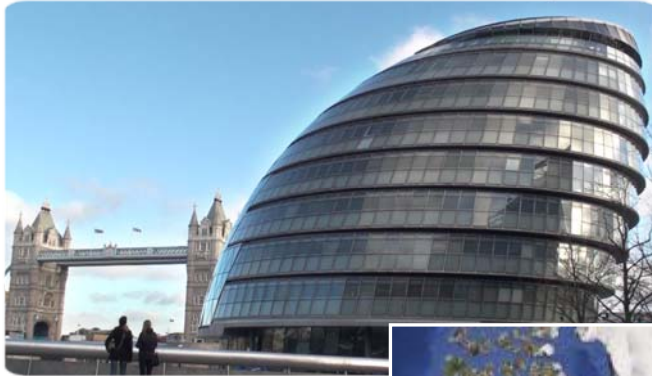
London, building retrofit
