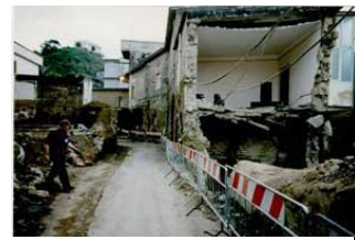
Landslide in Sarno 2001
