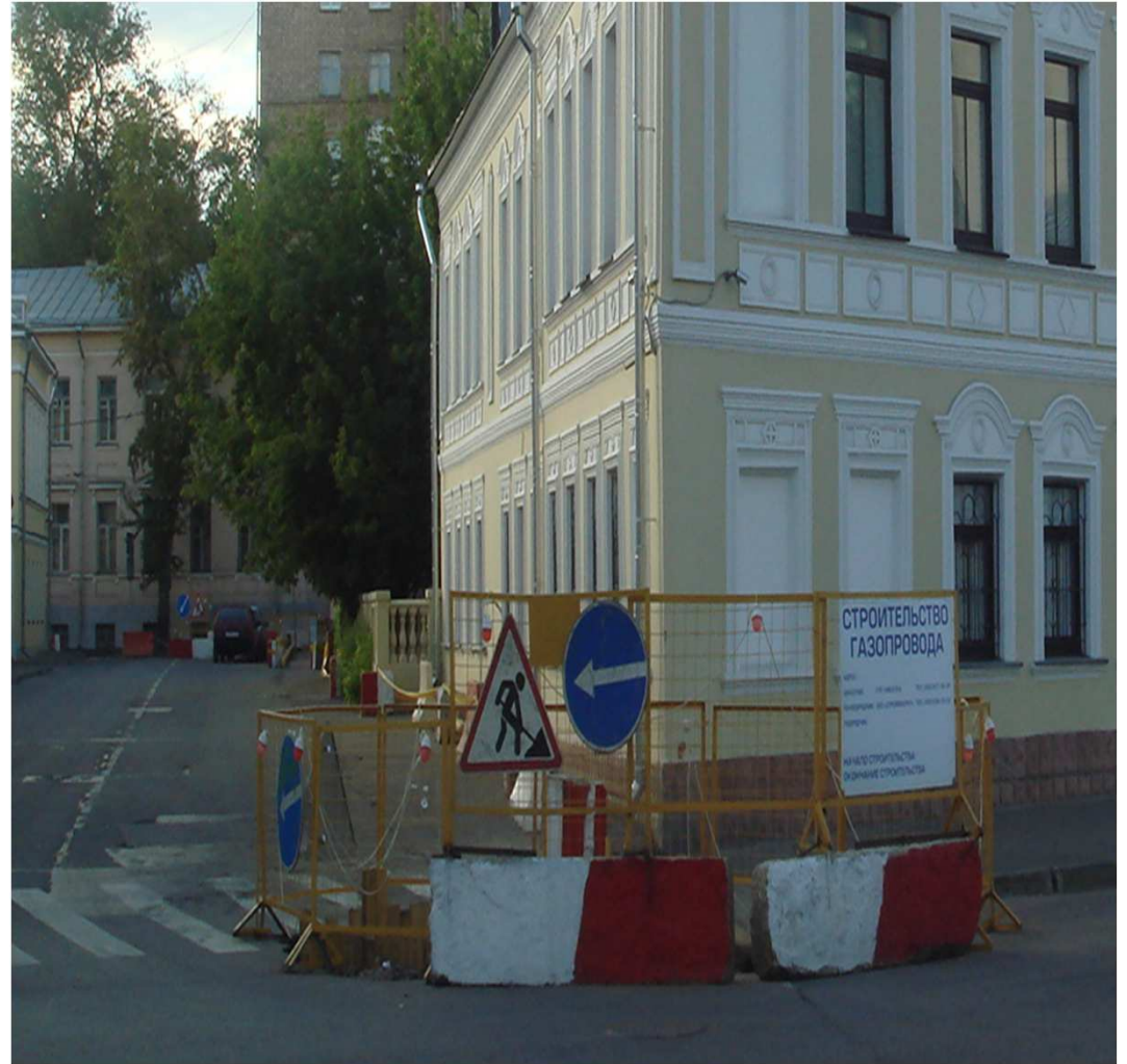
Sign: Construction of a gas pipeline, Central Moscow, 2009
