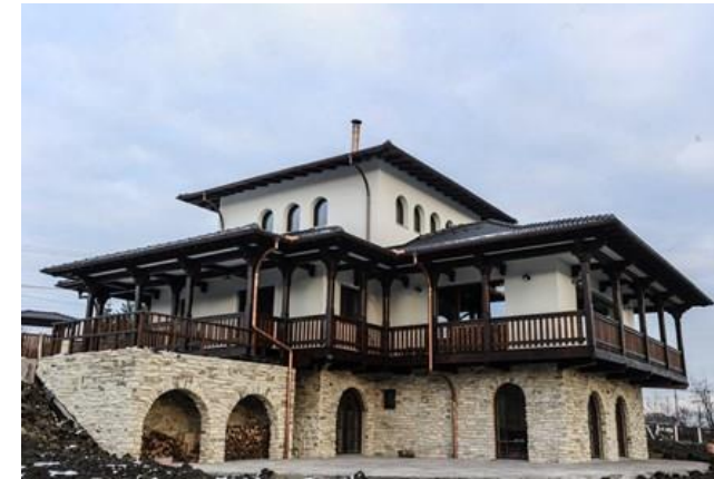
Single-family house, Passive House Plus in Romania ID: 4893
