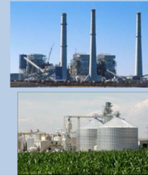
Downstream (refinery, power plants...)
