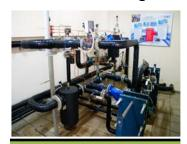
Regulating of heat supply depending on air temperature outside
