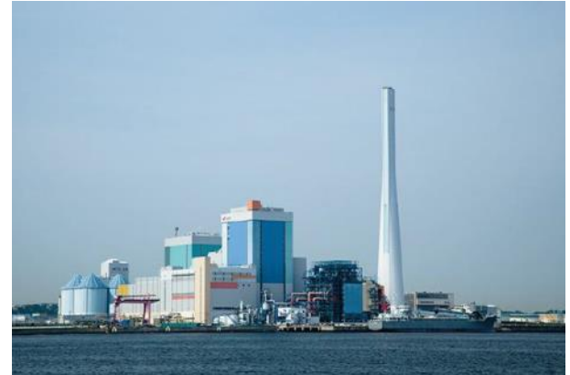
Japan: Isogo Power Station – Ultra Supercritical Technology (Courtesy of J – Power)
