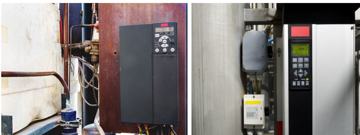
Figure 12. Frequency converters
