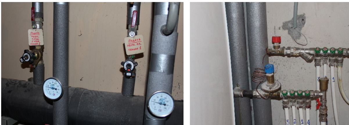
Figure 11. Example of balancing valves
