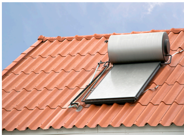
Passive solar system with flat collectors
