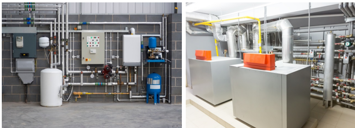
Figure 6. Examples of modern gas-fired boilers
